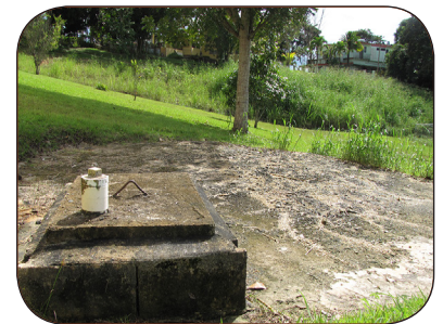
Keep septic tanks sealed.
